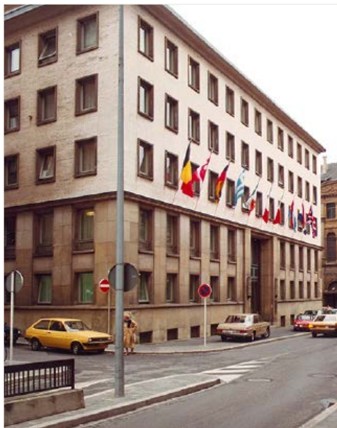
First ECA building, 29 rue Aldringen, Luxembourg
